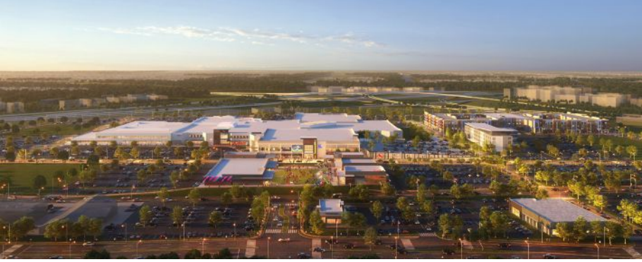
RUSSELL GLEN , a real estate development and investment firm, has redeveloped the former RedBird Mall in Dallas, Texas, into Shops at RedBird.
